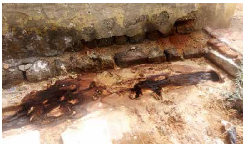
Effluents being taken to ETP through an open drain at a tannery in Peranambut
