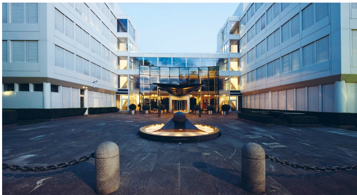
Glencore’s headquarters in Baar (Zug), Switzerland | © Mainrad Schade
