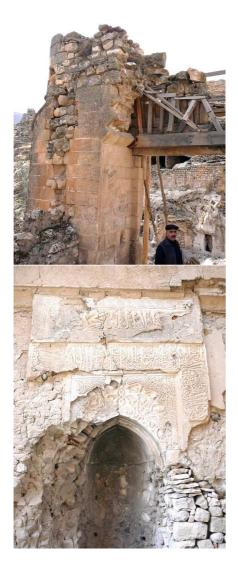
Photo 4: Hasankeyf, arch of an outer wall of the Büyük Saray. The arch is endangered from collapse. The building needs immediate conservation treatment.
